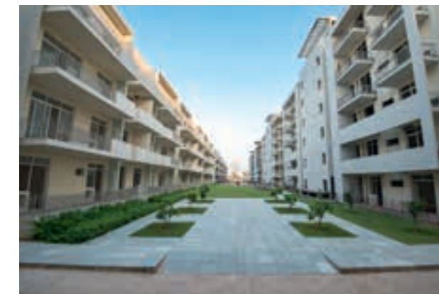
Over 200 families have already settled. 560 units are ready for possession out of 1150 apartments under construction
